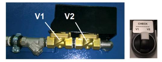
• Set the wet separator to maintenance condition. For that purpose the power supply for the control must be maintained, but the fan must be switched off. The door of the control housing must be opened.
